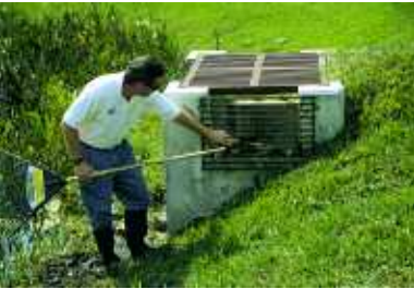
Clear or clean inflow/outflow structures.
